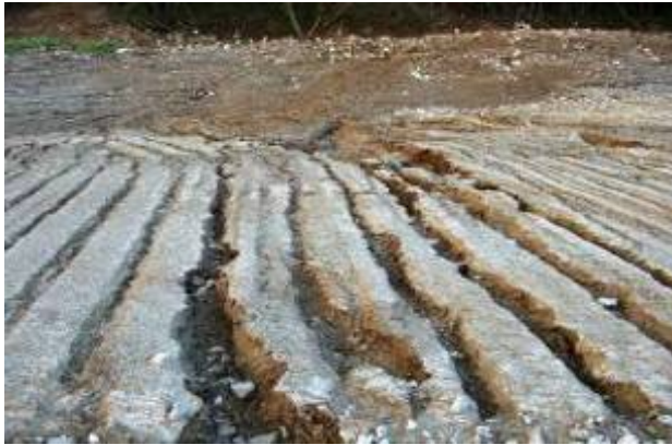
Strong erosion on topsoil deposited over the embankments
