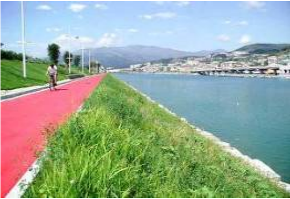
Genova Voltri, deep rooting plants installation by the seaside
