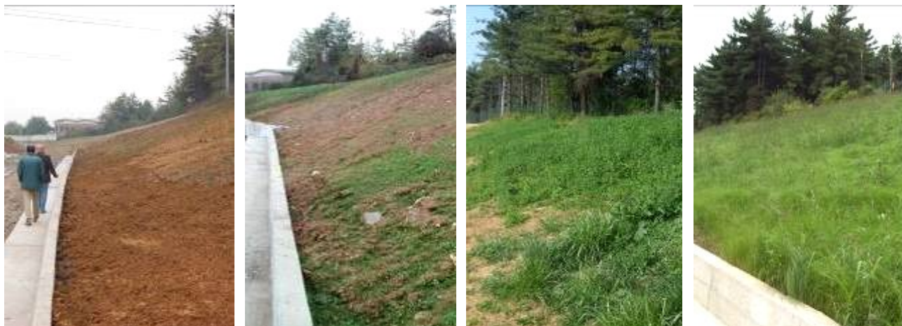
Villa d'Adda (northern Italy) – Development of PRATI ARMATI® vegetal blanket during 11 months from sowing
