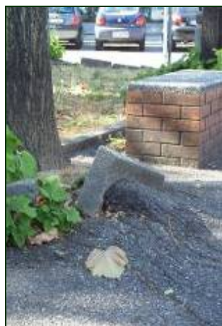
The roots of the trees are growing over time both in depth and diameter, causing swelling and fractures in the soil
