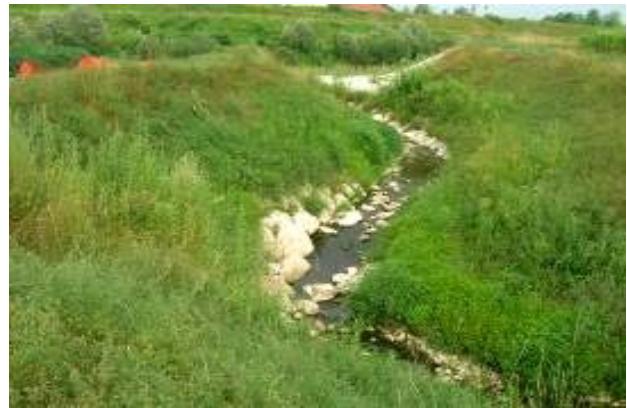
Same point of Meduna river with upper banks protected by PRATI ARMATI®
