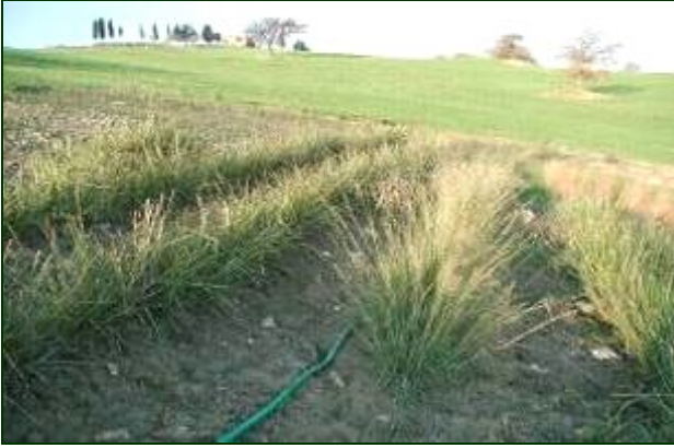
PRATI ARMATI® installation by Volterra (central Italy) on clay ground
