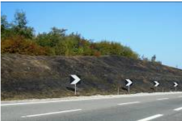
Italian motorway A6 - Old geonets remained barren for 15 years
