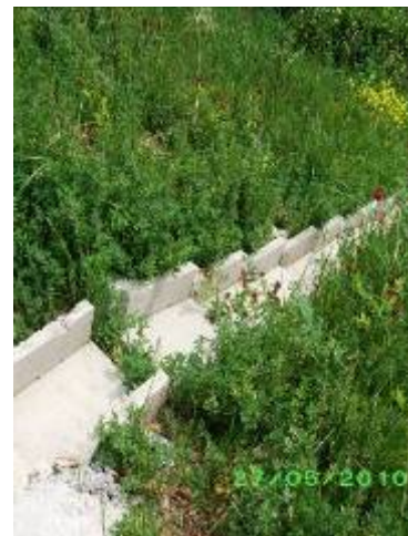
Drainage channels made with concrete modules on embankments protected by deep rooting herbaceous plants
