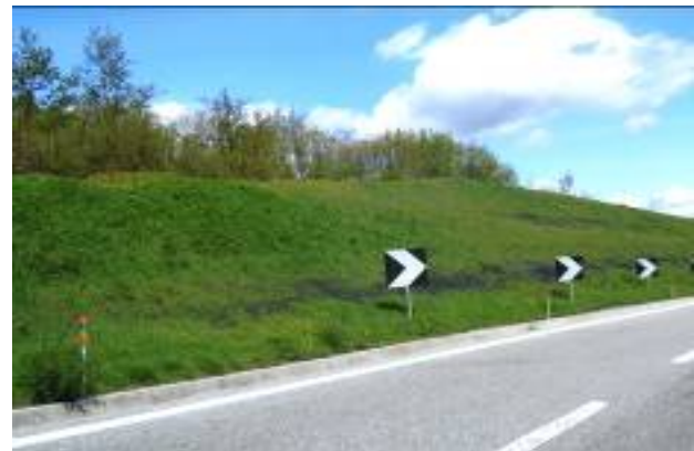
Italian motorway A6 after intervention with PRATI ARMATI®: erosion has been stopped, slope is renaturalized and black geonets are masked by a thick vegetal blanket
