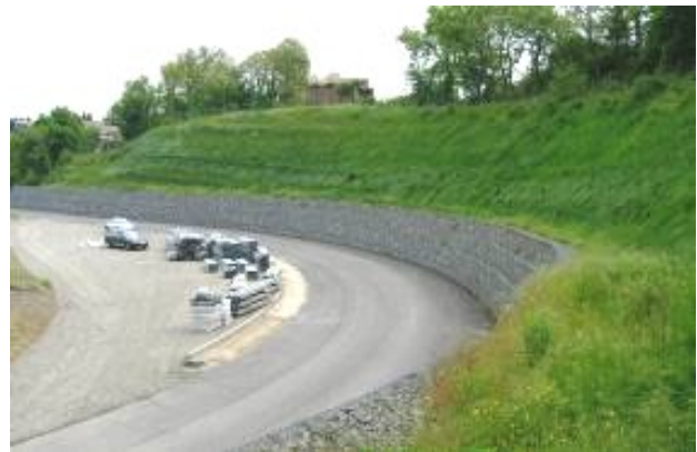
The new ring road with gabions protected upstream by herbaceous deep rooting plants
