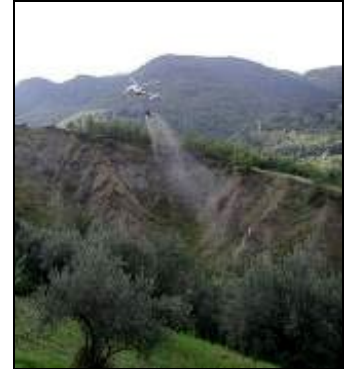
Hydroseeding by helicopters in large or inaccessible areas
