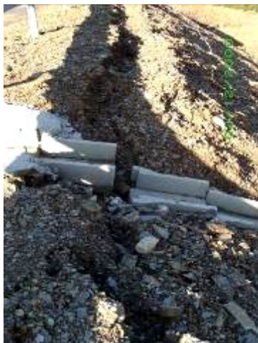
Yielding gutters made with tiles on road embankments
