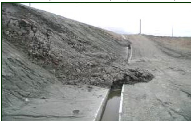
Land sliding due to excessive slope inclination and to erroneous collecting water, which resulted in a strong soaking clay soil
