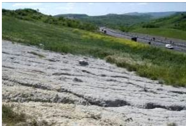
Motorway A1 Milan-Naples (Fabro): there is a clear separation between the area sown with PRATI ARMATI® and the original soil condition
