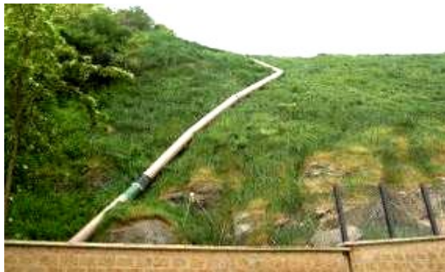
Orvieto (Central Italy) – The same area after PRATI ARMATI® installation. The erosion is stopped and the slope is renaturalized. The rockfall protection netting is hidden and protected from detachment: the deep rooting herbaceous plants anchor, thanks to their roots, the rockfall nets to the soil
