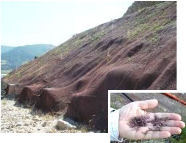
Plastic geonets 2 years after installation, degraded by atmospheric agents
