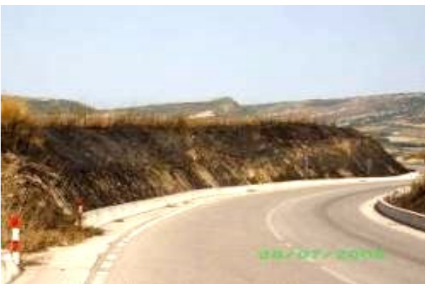
Florinas-Muros road (Sardinia): a slope treated with PRATI ARMATI® underwent a fire
