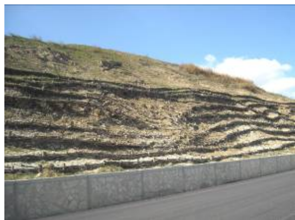
Collapsed anti-erosion installation based on wickerwork structures
