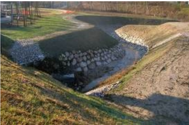
Meduna river (Northeast Italy): riverbank protection made with rock boulders in the lower part
