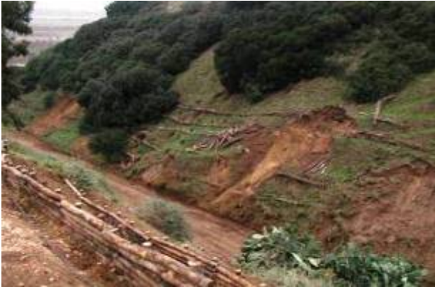
Municipality of Bernalda (Southern Italy) - A flood Collapsed the palisades in an untreated area
