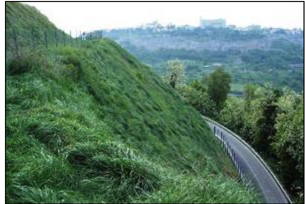
Hillside after PRATI ARMATI® installation. When the slope is steep, in case of heavy rainfall events, a major fraction of the rain runs over bedridden leaves, even when the vegetation is dried up, waterproofing the slope and protecting it from the erosive action of water.
