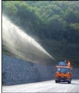
Hydroseeding in easily accessible areas
