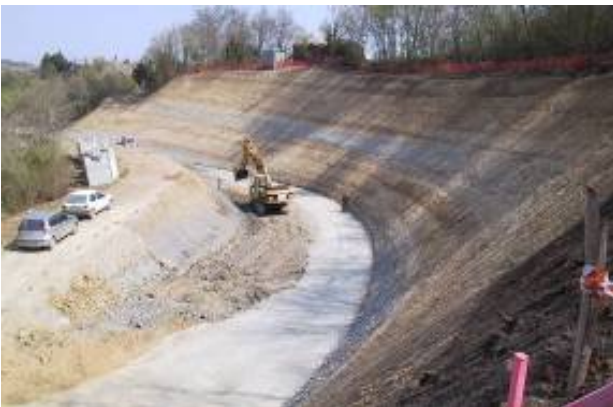
Castelviscardo (Central Italy), construction of the new ring road
