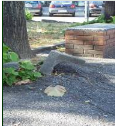
By the time the roots of the trees are growing both in depth and diameter, causing swelling and fractures in the soil
