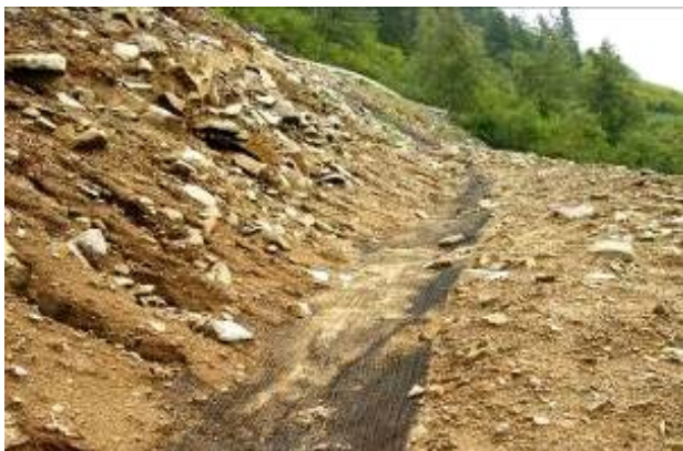
Oropa (Northern Italy) – Drain channels directly created on the ground as is
