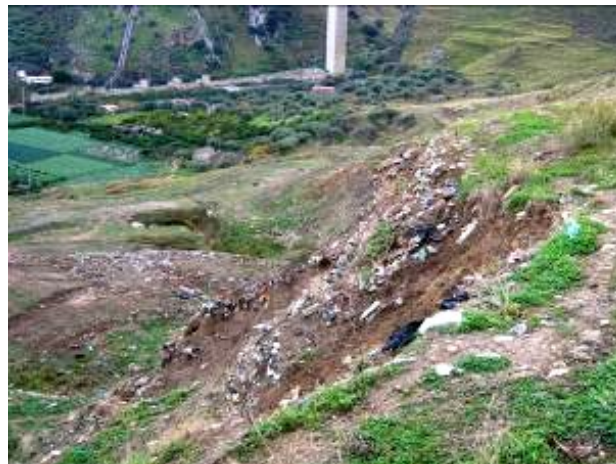
Example of a landfill slope
