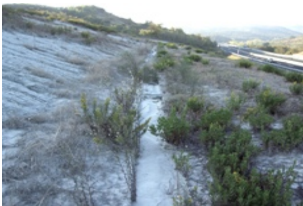
Motorway A1 Milan-Naples. Ditches were frequently clogged up and a continuous maintenance activity was necessary to keep them clean and efficient.
