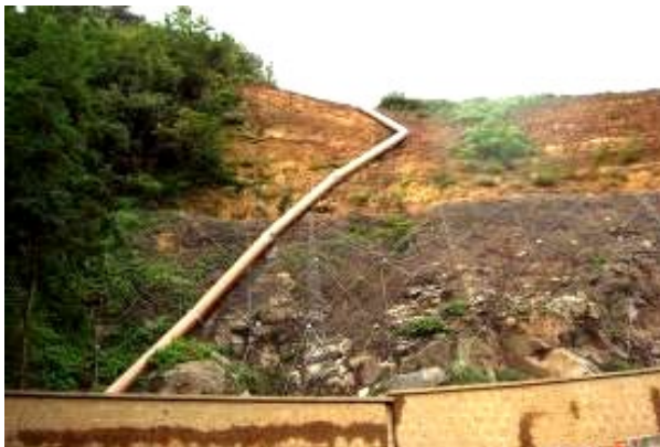
Orvieto (Central Italy) – Aggressive erosion on a slope protected only by rockfall protection netting.
