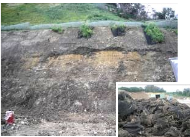
Collapse of an anti-erosion installation consisting of topsoil + plastics geonets + traditional hydroseeding + metal networks + deep nails
