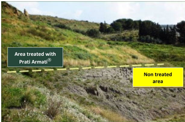
Sciacca (Sicily) - On a sample slope previously treated, the area left without vegetation is prone to cracks and crevices
