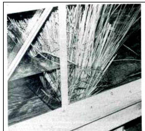
Filter effect of the vegetable blanket slowing down the flow of water
