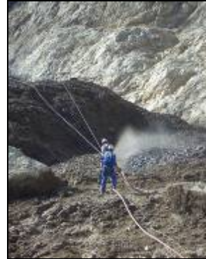
Hydroseeding by hosepipes handled by rock climbers
