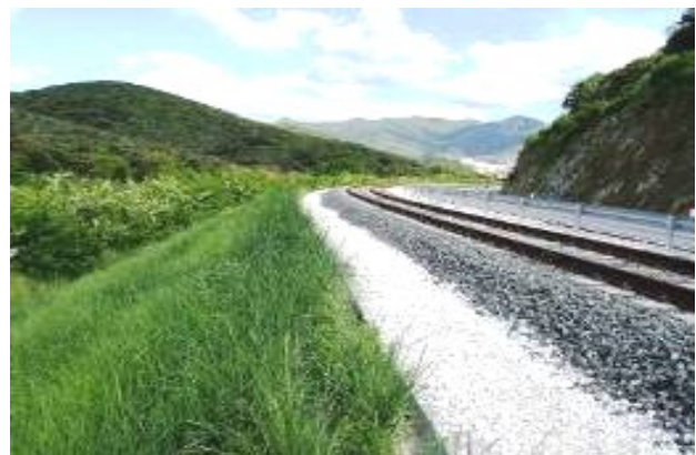
Tuscany. The railway embankments (50.000 m 2 ) after intervention with PRATI ARMATI® FOR EMBANKMENTS
