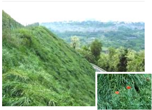
PRATI ARMATI® installation 2 years after sowing
