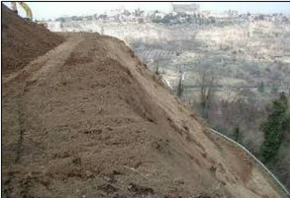
Orvieto (Central Italy) - Hillside before PRATI ARMATI® installation. The escarpment, without the protective vegetal blanket, is very exposed to the erosive action of water, especially in case of heavy rainstorm
