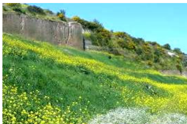
Typical aspect of a landfill protected with PRATI ARMATI®
