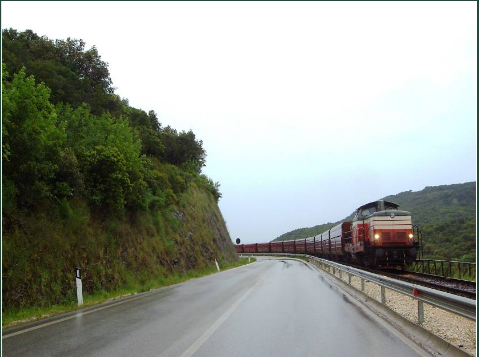
TUSCANY region, San Vincenzo (central Italy): railway works in San Carlo quarry
