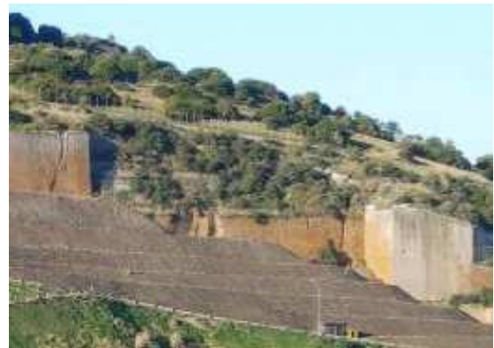
Figure 5: The MSW landfill Ozieri (Sardinia) in November 2005, before the intervention
