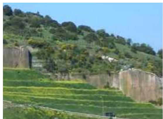
Figure 6: The MSW landfill in May 2006, after the intervention of re-naturalization with prati armati
